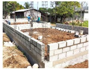
The project completed two adjoining classrooms of 20 x 26 feet each. There is a perimeter foundation supporting the walls and a 6-inch steel-mesh reinforced slab for the center floor area. Walls are made of cinderblocks with rebar reinforced concrete columns. The roof is made of zinc-coated sheet metal, built on a frame of 2 x 4 inch ushaped steel purlins.
